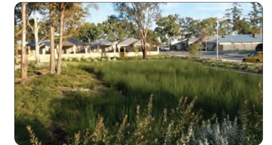
Vegetated drainage swale.
