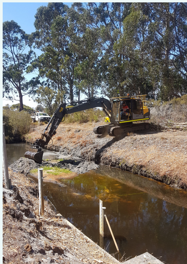
Removing the sand deposit in the weir pool at the Sleeman River sampling site, February 2019. This was done to improve the gauging station's ability to measure flow.
