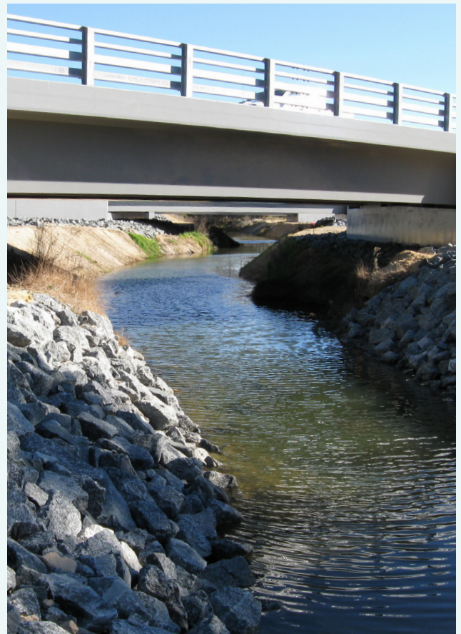
Stabilisation works undertaken on Mayfield Drain to help prevent bank erosion. This photograph was taken at the same location as the one of the previous page, June 2009.
