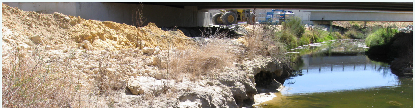
Mayfield Drain at the Forrest Highway bridge. Note the erosion and undercutting of the bank on the left side of this photograph, March 2009.
