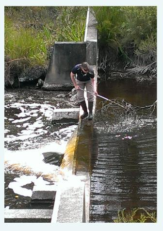
Cleaning debris off the weir at the Kalgan River sampling site. High flows can wash debris onto the weir, which impacts flow measurements, November 2015.
