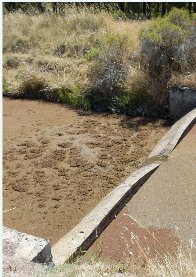
High nutrient concentrations encourage macrophyte growth. Here the drain is completely covered by macrophytes, December 2014.
