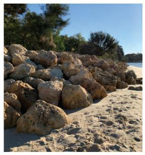
Image 19. Example of rock revetment coastal protection works.
