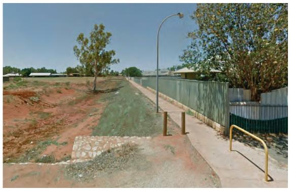
Image 29. Example in Kennedy Street, South Hedland of an open swale drain adjacent to residential lots with a side pathway. This principle is envisaged for the drainage corridors in the structure plan where provision of a pathway is considered appropriate, to increase pedestrian connectivity and accessibility to the foreshore. (Source: Google maps street view, 2020)
