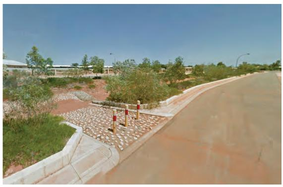
Image 28. Example in Gannet Street, South Hedland of rock pitching and kerb break to allow stormwater to discharge from road into the roadside open drain.(Source: Google maps street view, 2020)
