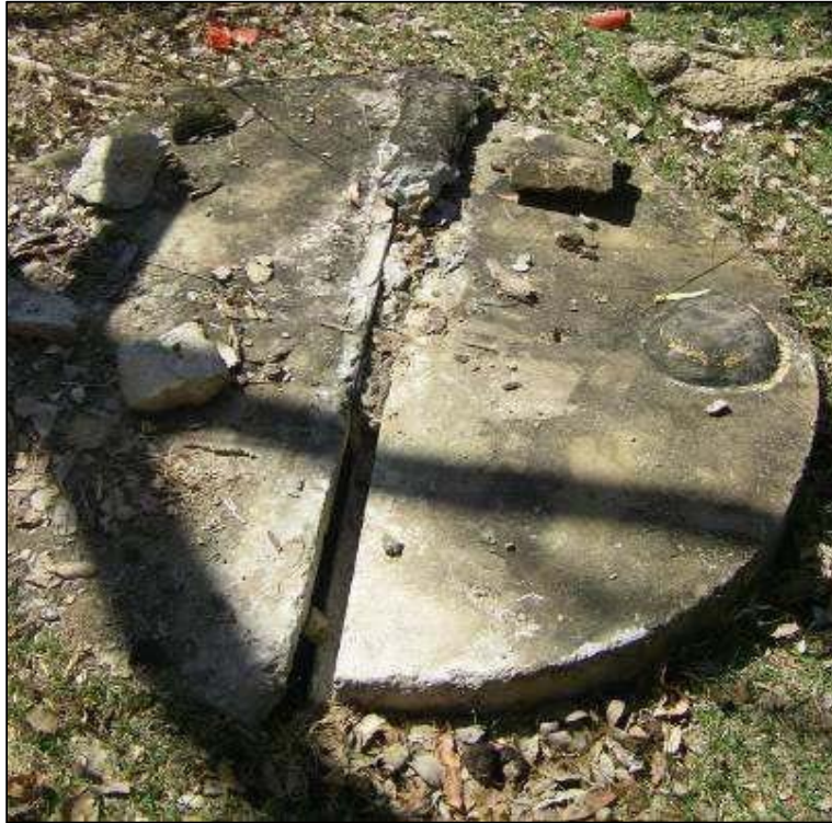
Figure 8 – Septic tanks at the rear of SL-lot 10
