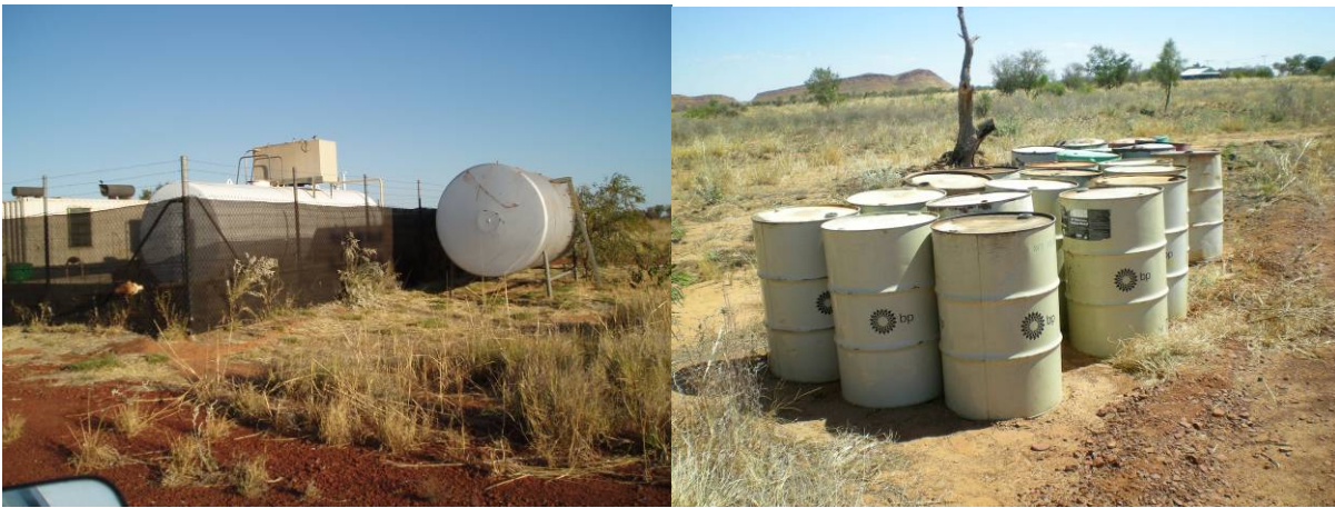
Figure 15 - Power station: fuel storage tank and empty diesel drums outside of generator compound
