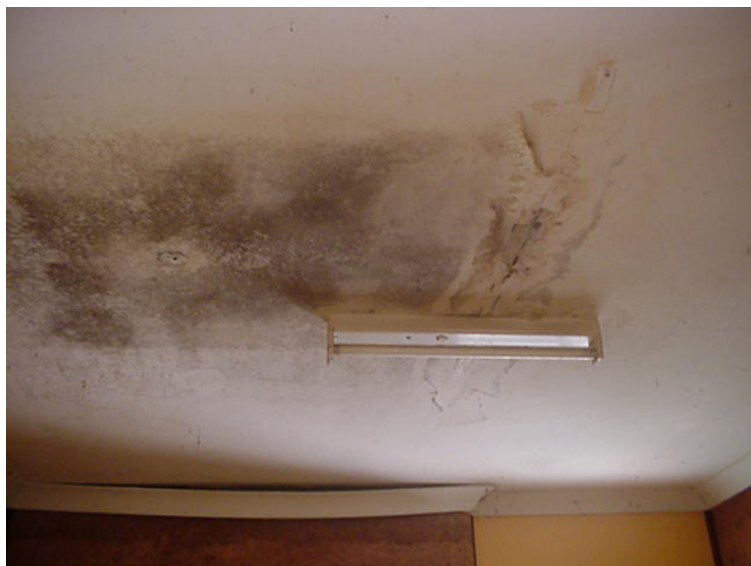
Figure 2 - Buckled cornice & water damage to ceiling in kitchen area due to housing design/construction and environmental conditions (source: Shire EHO 2003)
