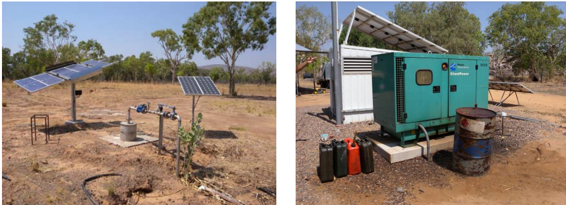
Figure 3 & 4 Solar powered bore (left) and solar/diesel hybrid power generator (right).
