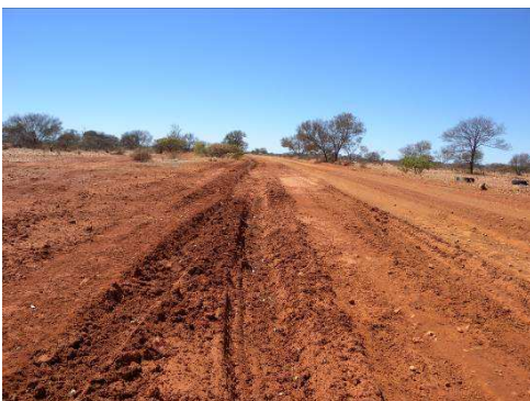
Figures 11 and 12: The airstrip road showing surface wear
