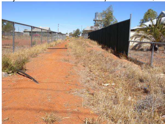
Figures 4 and 5: Overgrown drainage swales.
