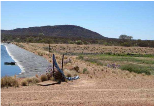
Figure 9: Primary wastewater pond lined and unlined secondary pond
