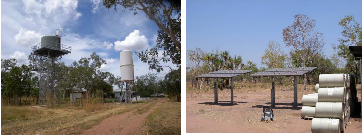
Figures 4 & 5 - Elevated water tanks (left) and solar/diesel hybrid with build up of empty diesel drums (right).
