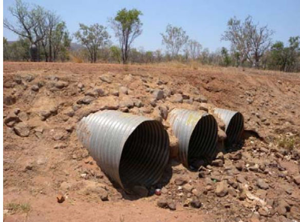
Figure 7 & 8 - Access road into Wijilawarrim (left) and culverts under access road (right).
