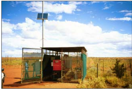
Pump station for the water bore
