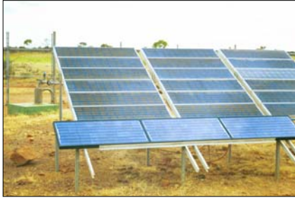
Solar power operation of the water bores.
