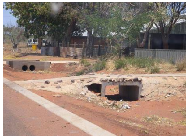
Figure 8 - Constructed Culverts over drainage channels
